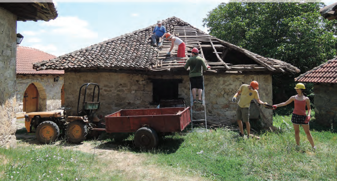
Removing and storing the roof tiles from the cellar of Jevka Aleksić.
