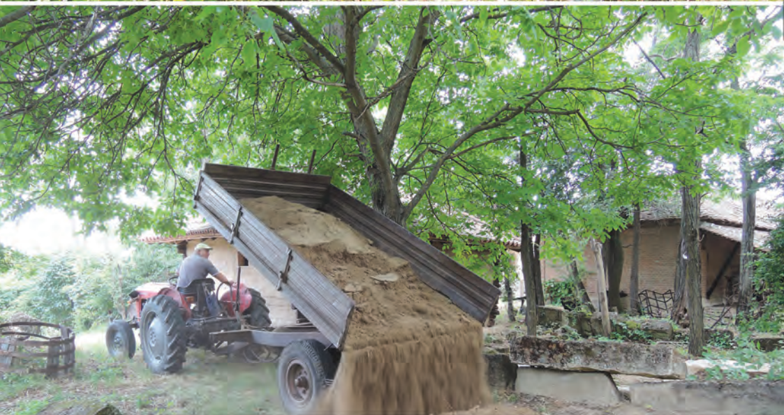
Harvesting the earth / mud "muljak" from the former site of the Rajić brick factory near the Timok River, and bringing it to the construction site.
